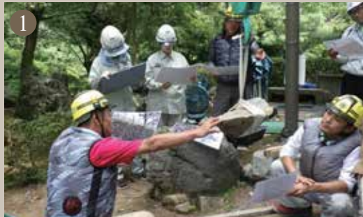
1 We are specifying the original locations of the stones from the collapsed walls.
