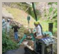
Recovery and storage of collapsed stones
